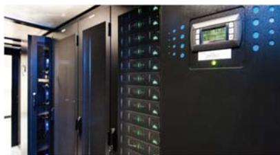
A computer room air conditioning (CRAC) unit is a device that monitors and maintains the temperature, air distribution and humidity in a network room or data center. CRAC units are replacing air-conditioning units that were used in the past to cool data centers. According to Industrial Market Trends, mainframes and racks of servers can get as hot as a seven-foot tower of powered toaster ovens, so climate control is an important part of the data center's infrastructure.
